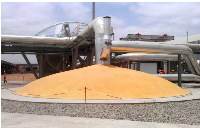
Rock bed based thermal energy storage in Ait Baha, Morocco, operating in a concentrated solar power plant
